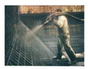
When handling spray concrete, the specially mixed material is fed from the concrete mixer truck into the pump's storage tank and is then applied to the surface through special spray equipment. Depending on the strength and application thickness needed, an accelerator can be metered into the sprayer to shorten the curing time of the concrete.
