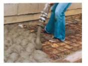
When concreting, the concrete is delivered into the shuttering, compressed, levelled and then possibly re-treated. The concrete can be conveniently applied thanks to the modern technology of the S-transfer tube.
